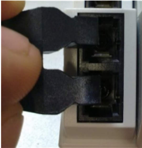
Figure: Blind plugs in unused sockets
